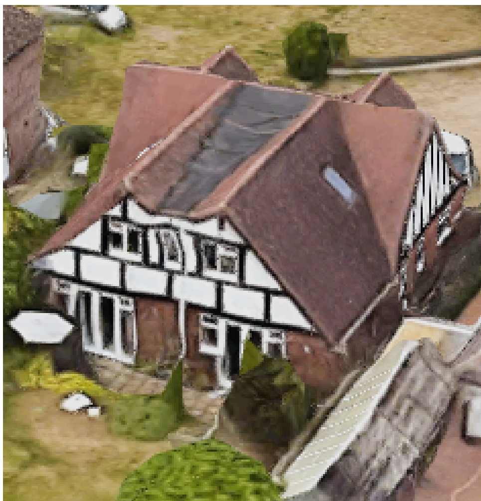
Figure 3: Example of a 2-span roof form approximately 60m to the west (no.8).
